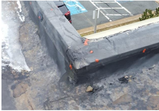
Photo B.43 – Sealant patches at flashing screw holes
