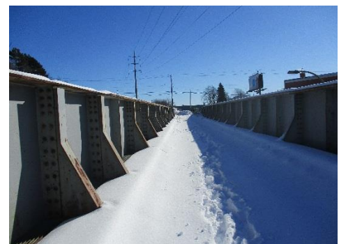
Figure 2: Top of deck on day of inspection.
