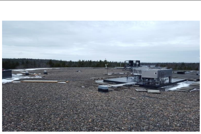
Photo B.5 – Roof surface, west facing.
