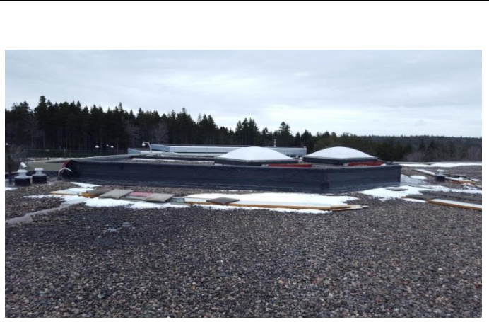
Photo B.6 – Roof surface, southwest facing.
