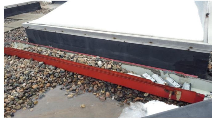
Photo B.38 – More flashing secured with ballast.
