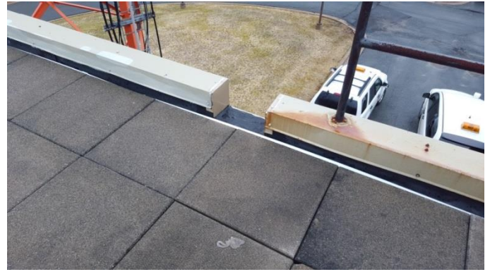
Photo B.20 – Scupper on north side of roof.
