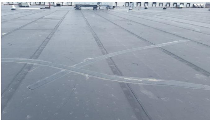
Photo B.47 – Overlapping patches, mid-roof.
