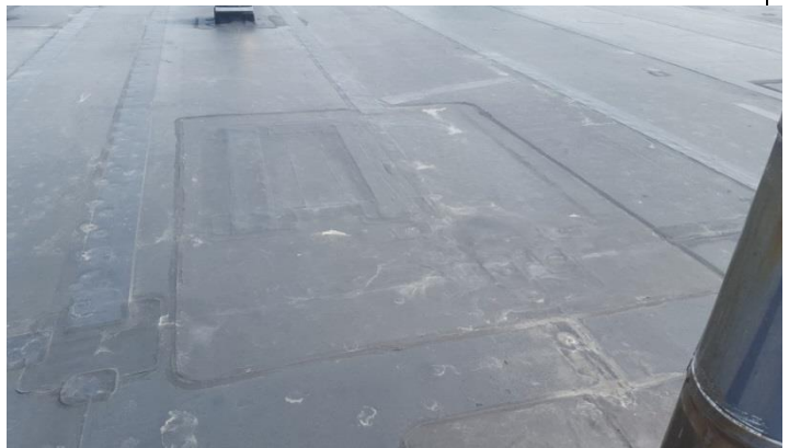
Photo B.6 – Roof surface patch at HVAC removal.
