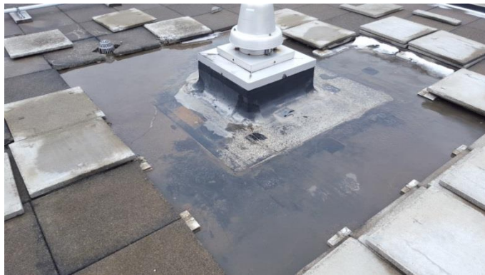
Photo B.21 – Membrane patches around vent.
