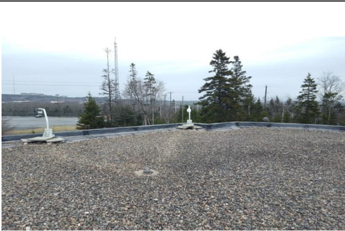
Photo B.1 – Roof surface, northeast facing.
