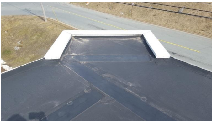
Photo B.15 – Parapet at northwest corner.
