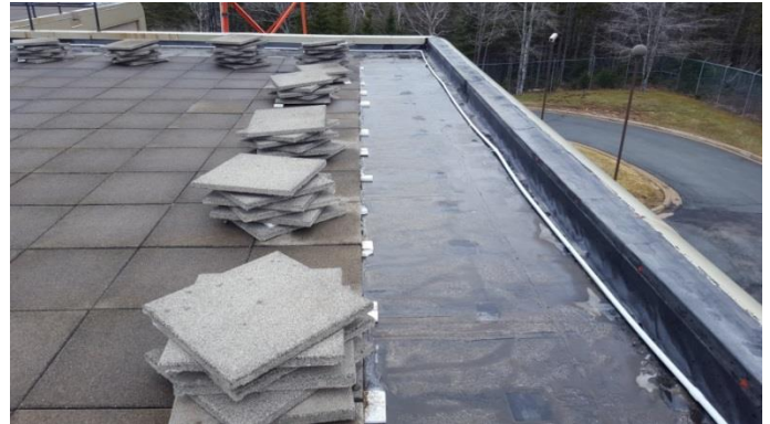
Photo B.14 – Stacks of pavers near roof edge.
