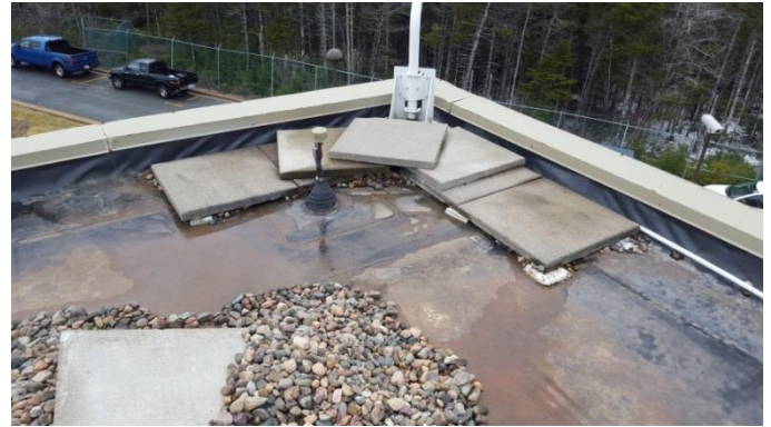
Photo B.32 – Light fixture and boot flashing (SW).
