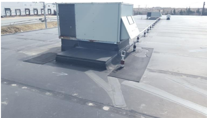
Photo B.51 – Secondary HVAC unit pipe supports.
