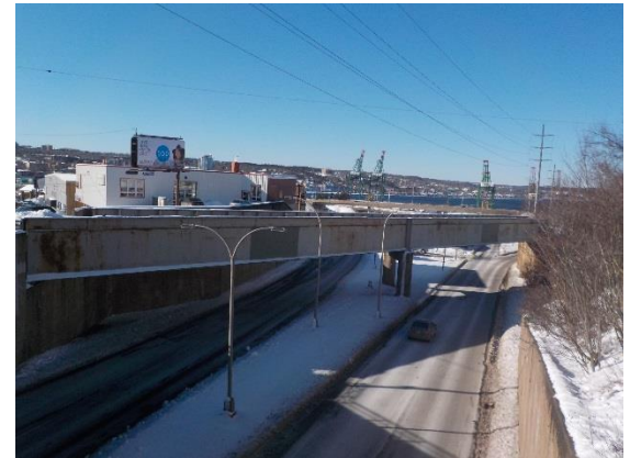
Figure 1: Former CN Railway Bridge.
