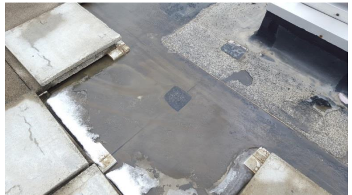
Photo B.22 – Membrane patches around vent.
