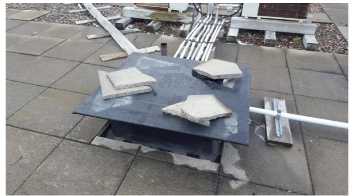
Photo B.24 – Ballast securing temporary curb cover.
