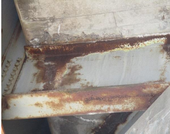
Figure 15: Spall on concrete deck above floor beam.
