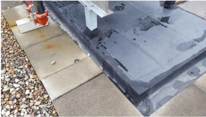
Photo B.31 – New equipment curb (no issues).
