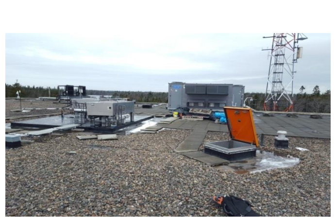
Photo B.4 – Roof surface, northwest facing.
