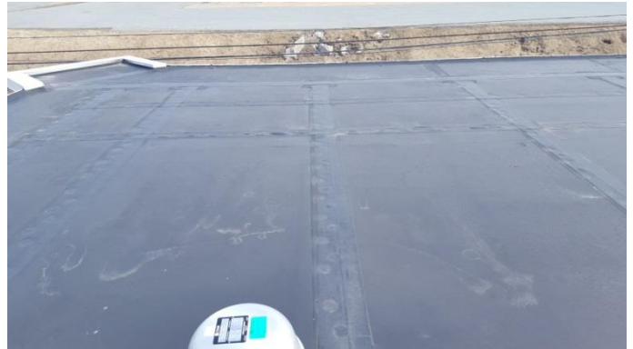
Photo B.14 – Typical mechanical attachment seam.
