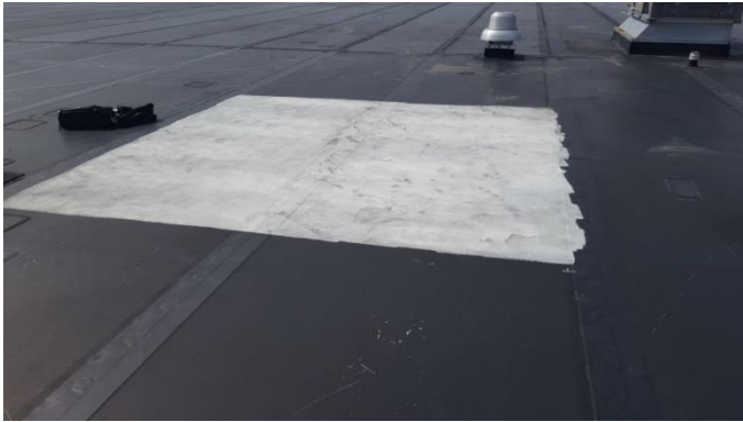
Photo B.43 – Reflective coating test near roof hatch
