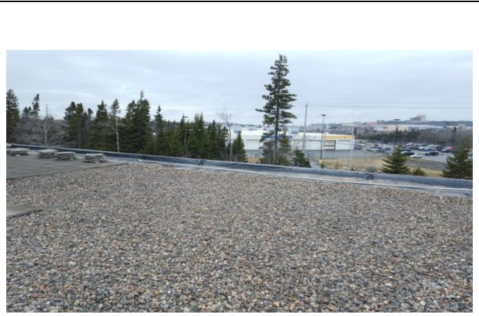
Photo B.2 – Roof surface, north facing.
