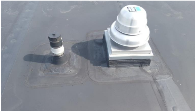
Photo B.13 – Flashing boot at capped stack.
