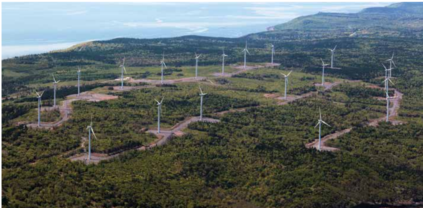
Completed in 2010, the Digby Neck Wind Farm supplies up to 10,000 homes. Photo courtesy of Nova Scotia Power Inc.
