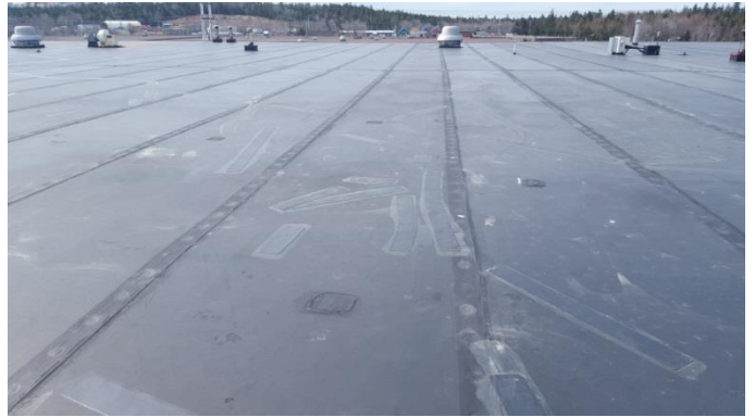
Photo B.44 – Overview of patches near hatch.
