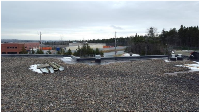
Photo B.7 – Roof surface, south facing.
