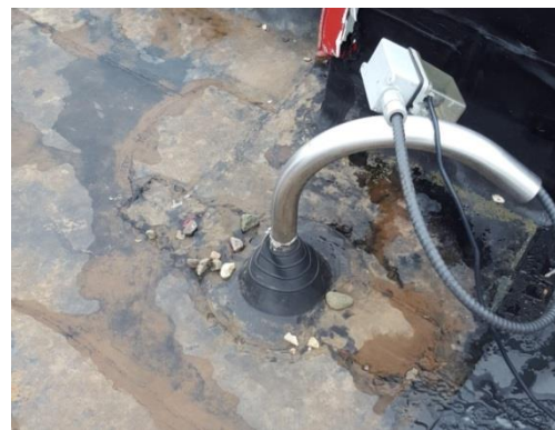
Photo B.42 – Penetration boot (good condition).
