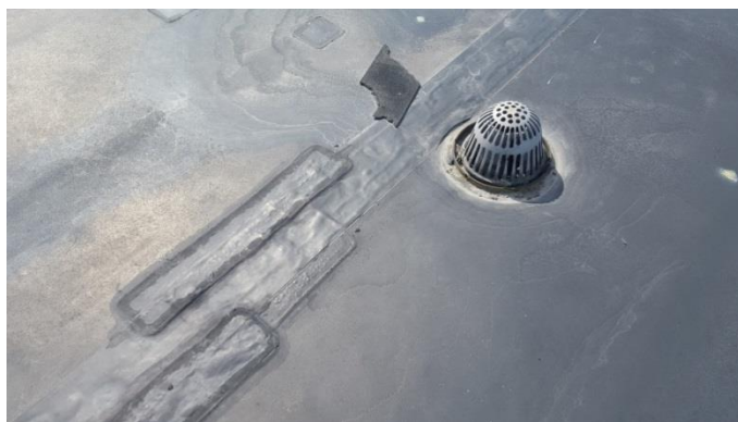
Photo B.23 – Patching adjacent to a roof drain.
