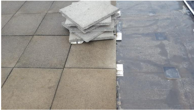
Photo B.13 – Paver mounting detail (EPS strip).
