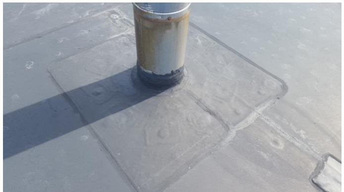
Photo B.4 – Penetration flashing, west side.
