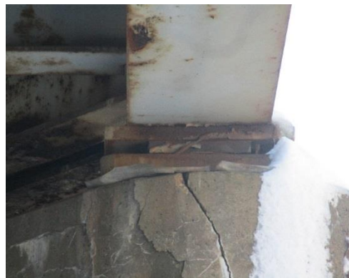
Figure 11: Overhang of pier bearing assembly.
