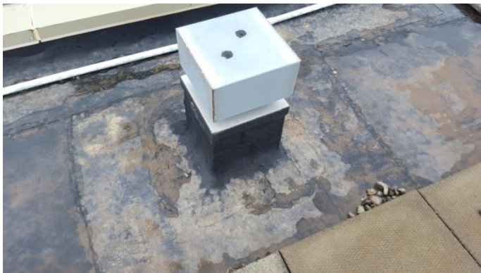
Photo B.27 – Typical curbed vent penetration.
