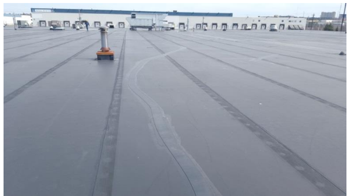
Photo B.46 – Long patch cover strip mid-roof.
