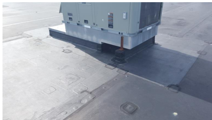
Photo B.21 – Membrane repair around HVAC unit.
