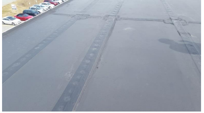
Photo B.2 – Roof surface, west edge, taped seam.
