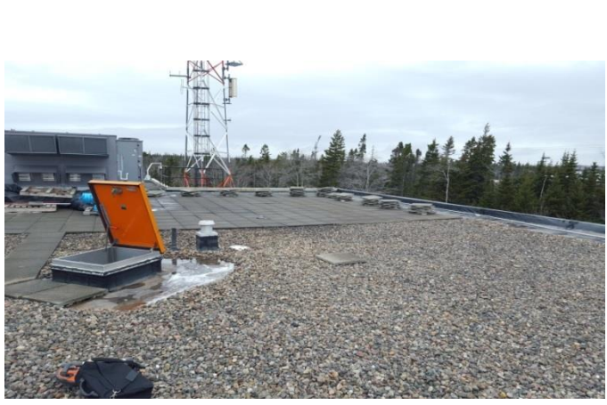
Photo B.3 – Roof surface, north facing.
