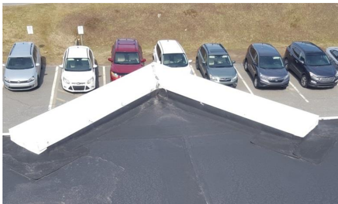
Photo B.9 – West facing parapet.
