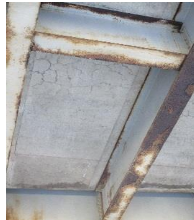
Figure 14: Floor beam and stringer condition.
