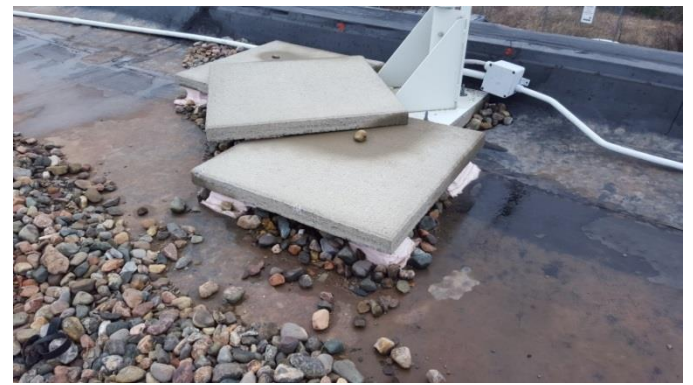
Photo B.10 – Precast paver mounting at fixture.
