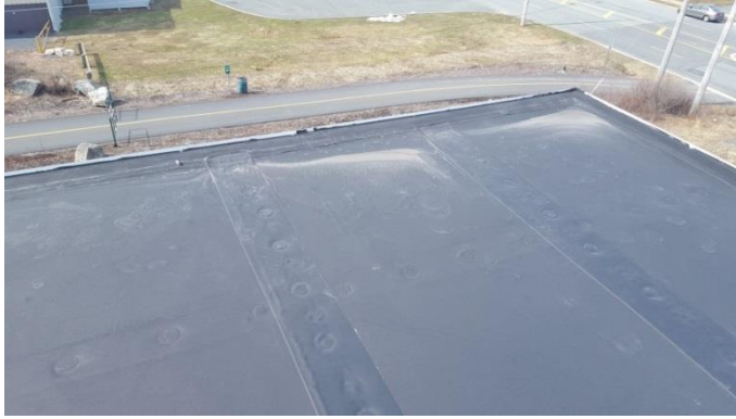
Photo B.1 – Roof surface, southwest corner.
