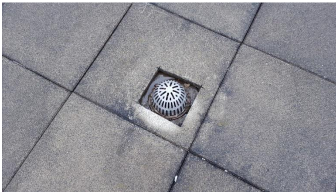
Photo B.15 – Opening in pavers for drains.
