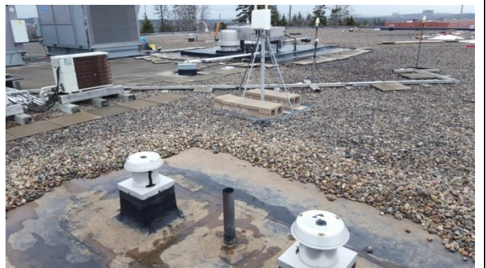
Photo B.30 – Note equipment on timber sleepers.
