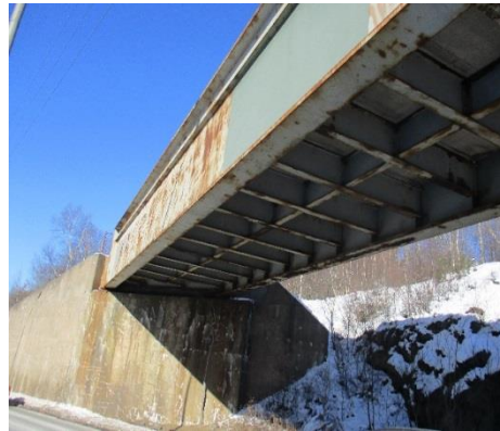
Figure 13 - Typical girder condition
