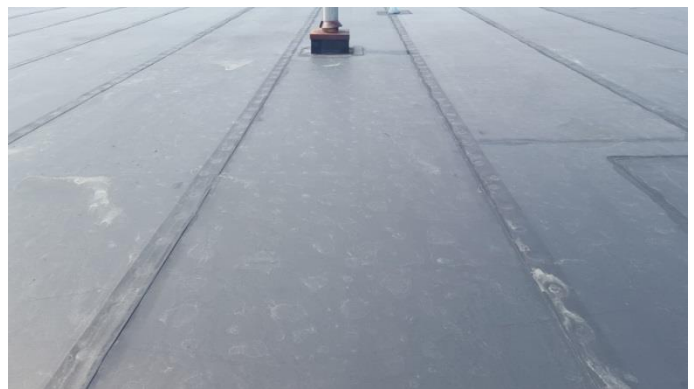
Photo B.30 – Typical original seams, mid-roof area.
