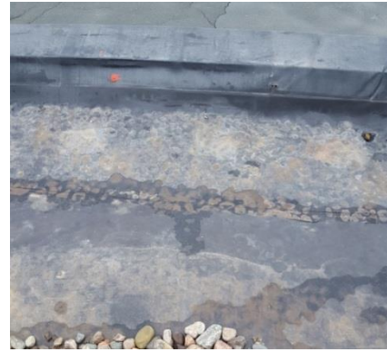
Photo B.44 – Typical screw hole without sealant.
