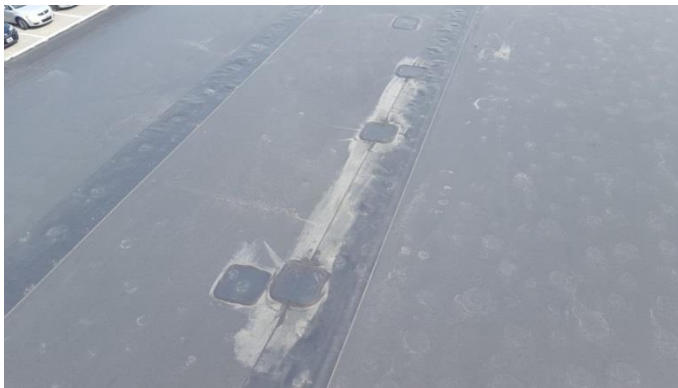
Photo B.3 – Roof surface, west edge, taped seam.
