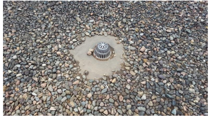
Photo B.8 – Typical roof drain.
