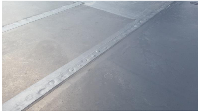
Photo B.20 – Fasteners sitting proud of substrate.
