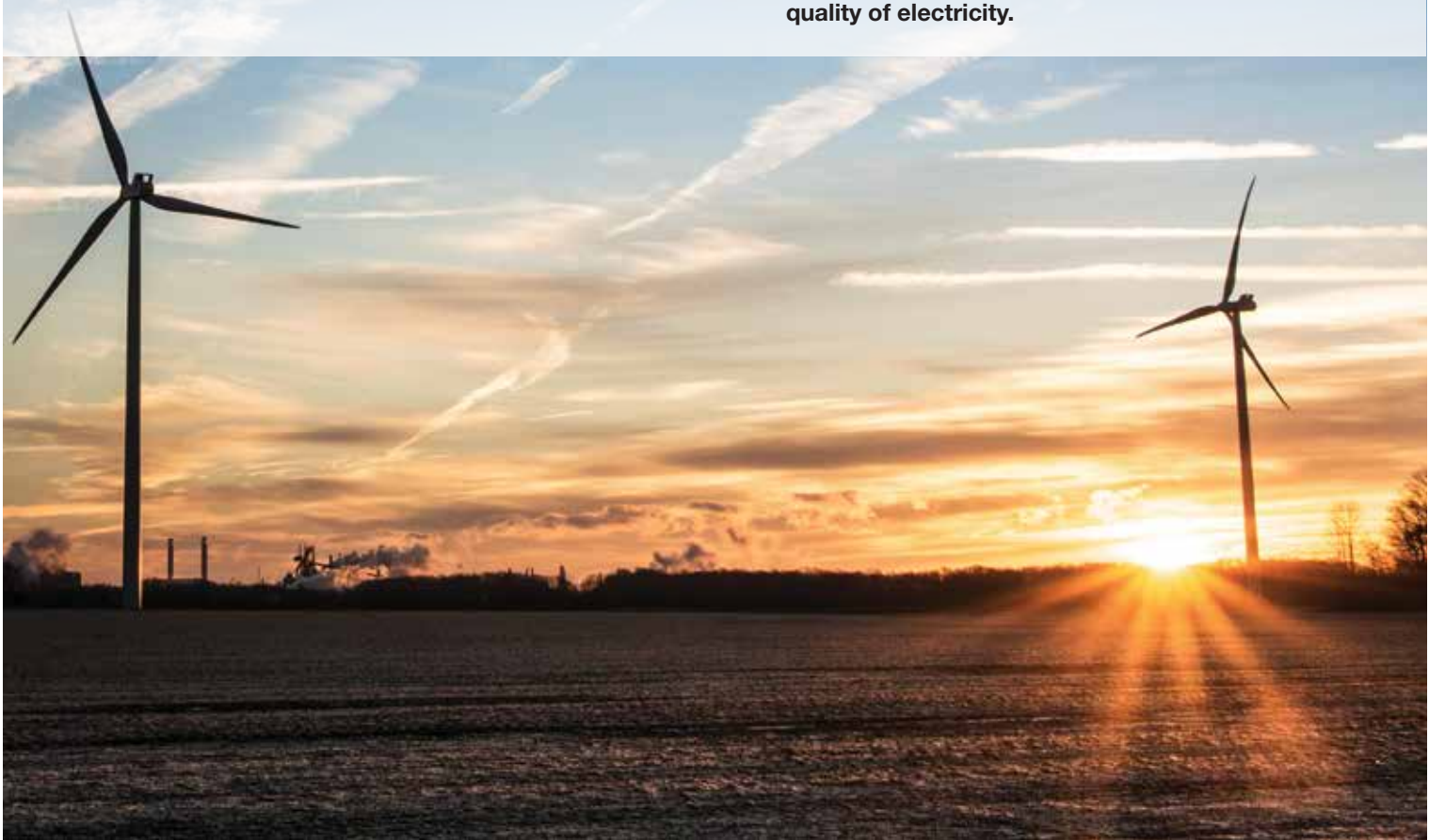
Capital Power Corporation’s 105 megawatt Port Dover and Nanticoke Wind project is located in Haldimand and Norfolk Counties, Ontario. The project, which began commercial operations in November 2013, features 58 Vestas V-90 turbines. Photo courtesy of Capital Power Corporation.
